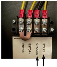
The two remote start leads from the Automatic Transfer Switch are connected to the two terminals marked GROUND & START. The WIRE in terminal GROUND is battery negative and the wire in the terminal labeled START is your remote start lead. Closing these two leads together will signal the DSE 7310 MKII to go into an autostart mode and start up the generator.
