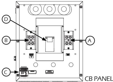
**A - Neutral Lugs**, These neutral lugs are isolated from ground and provided for you to connect your neutral wire from the transfer switch. The lugs will handle wire sizes #1 AWG TO 300 MCM and should be torqued to 250 in. lbs.
